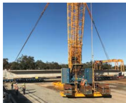
Preparing to lift one of the beams into place along the Northern Section of NorthLink WA.
